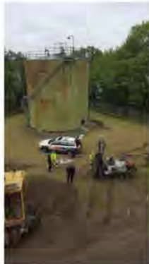
In situ installation - Motala
